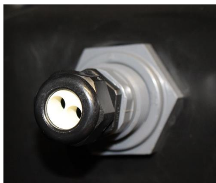
Double gland for level sensor and high-level float
