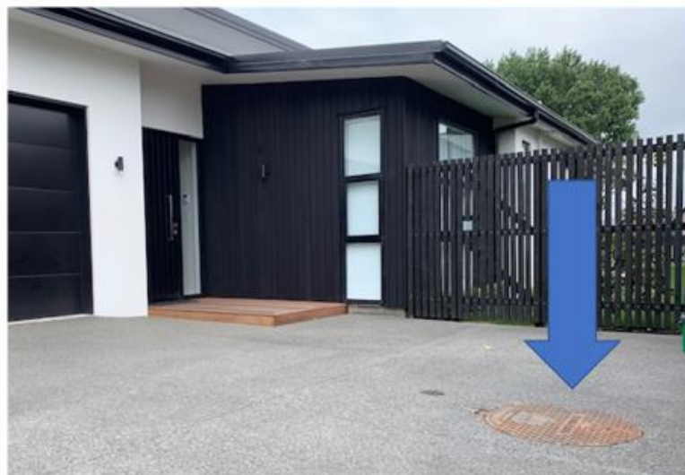
Example of tank in driveway with metal manhole lid
