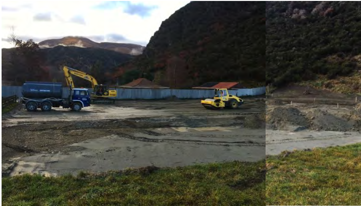
Photo 1: Showing rolling of the placed fill material underway
