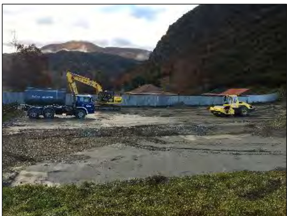
Photo 3: Looking North from Lot 12 towards Lot 13 where earthfill placement and compaction was occurring.
